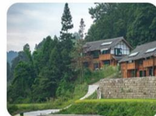
3: 民宿供电 Power supply for homestays
